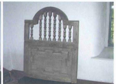
160 ORIGINAL FRONT ENTRY GATE
