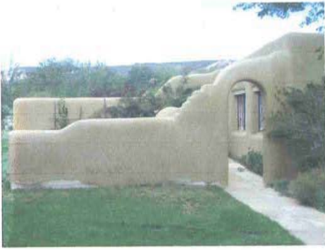
194 GARAGE S PATIO
