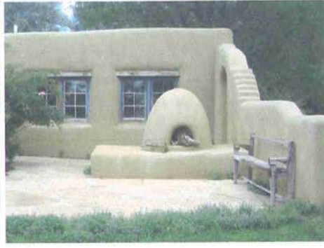
195 GARAGE S PATIO
